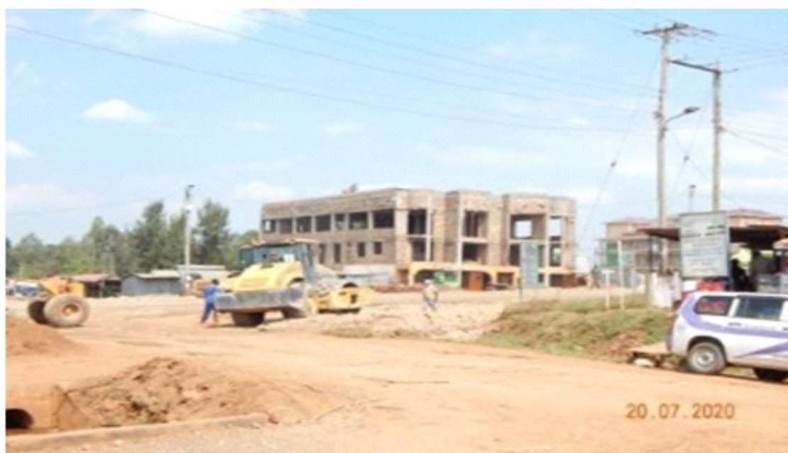
Figure : Ongoing road expansion in Awendo Municipality
