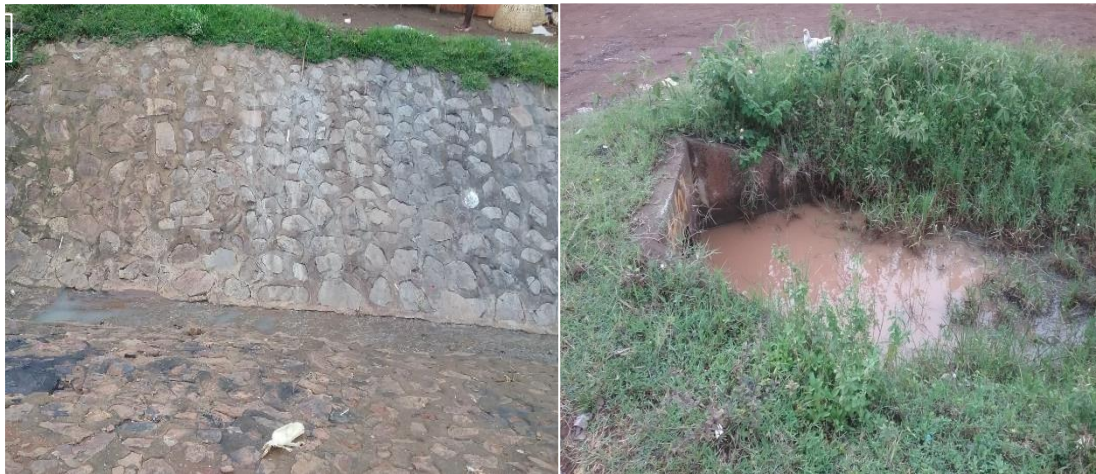
A Paved Storm Water Drainage Channel
