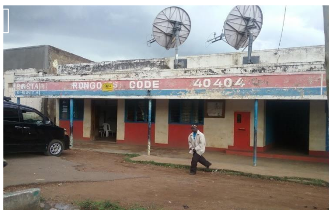
Figure 39: Rongo Post office
